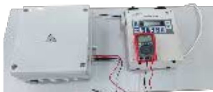
Testing start-up protection equipment and control equipment for suitability EM-PPAAU
